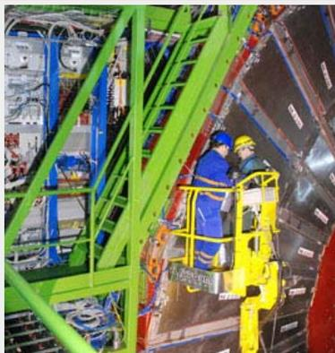
Replacing the bushings, water is being drained by 2 ZEC workers and Dan Wenman, an engineer from PSL (by Richard Breardon)
